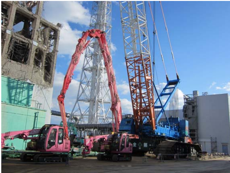
⑬- 1 Large size heavy machine for dismantling Jan. 14, 2012 photo by TEPCO staff
