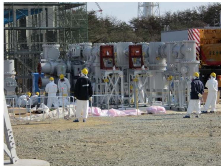
⑦-11 Construction of new switch station Jan.10, 2011 photo by TEPCO staff
