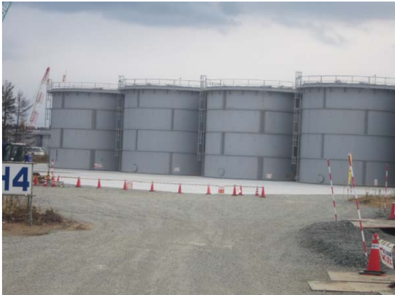
⑧-1 Tank array at H area Jan. 9, 2012 photo by TEPCO staff
