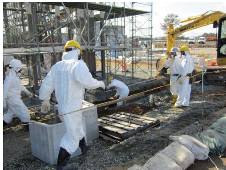
⑦-9 Construction of new switch station Jan.10, 2011 photo by TEPCO staff
