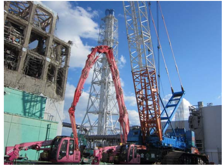
⑬- 2 Large size heavy machine for dismantling Jan. 14, 2012 photo by TEPCO staff
