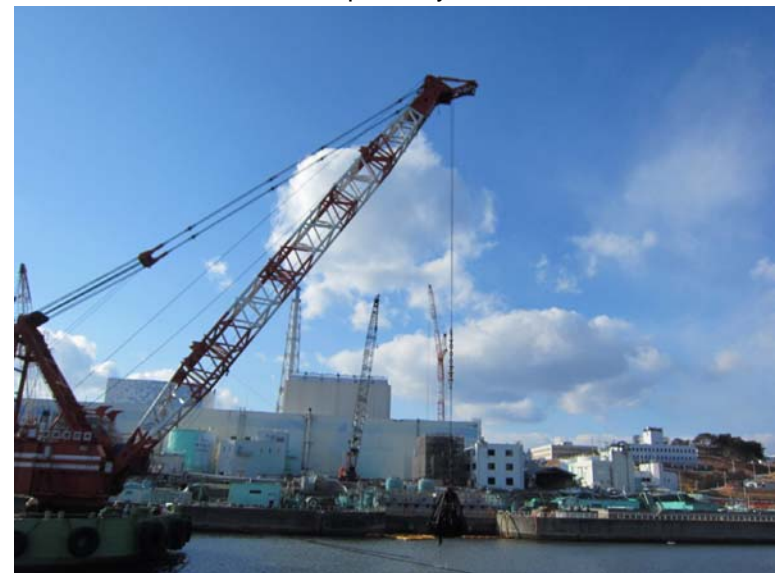
③-7 Removal of obstacle by the floating crane (from east breakwater)
