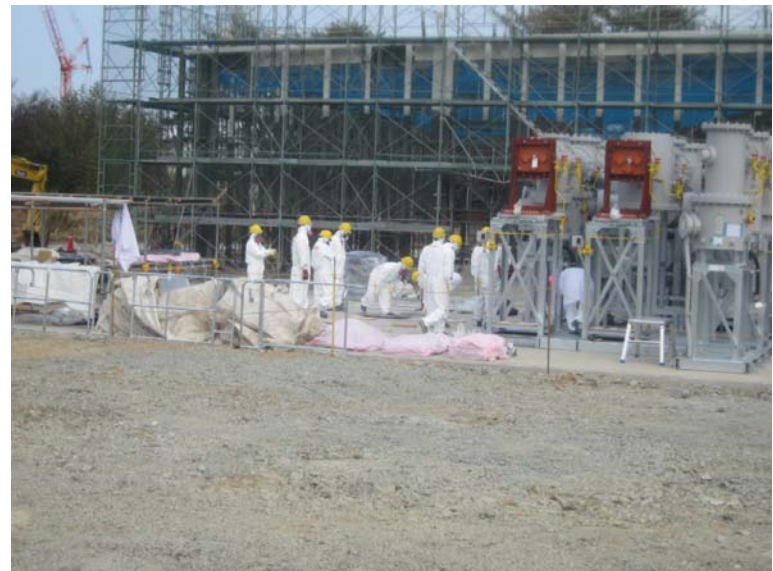
⑦-4 Construction of new switch station Jan. 9, 2011 photo by TEPCO staff
