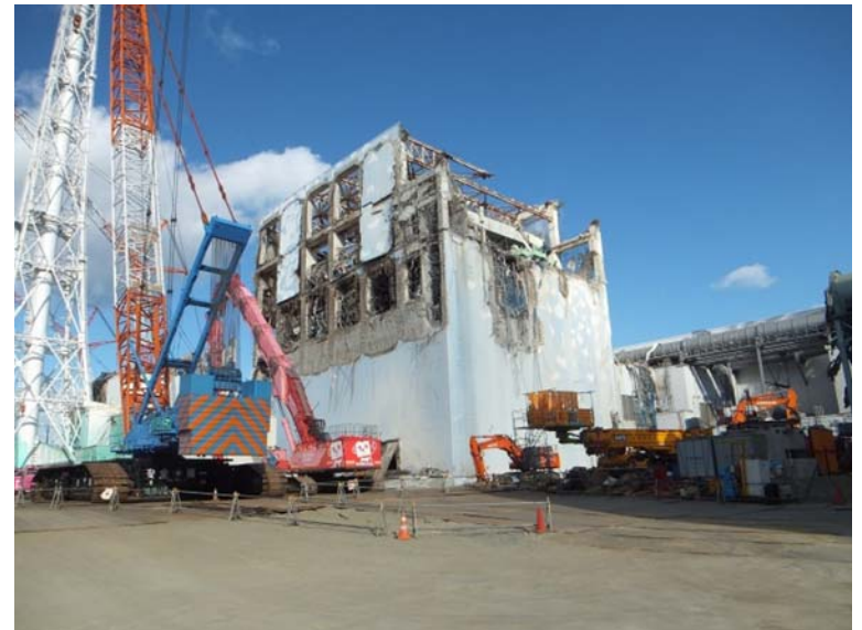
①-8 Removal of debris on the upper side of Unit 4 Reactor Building (after work)
