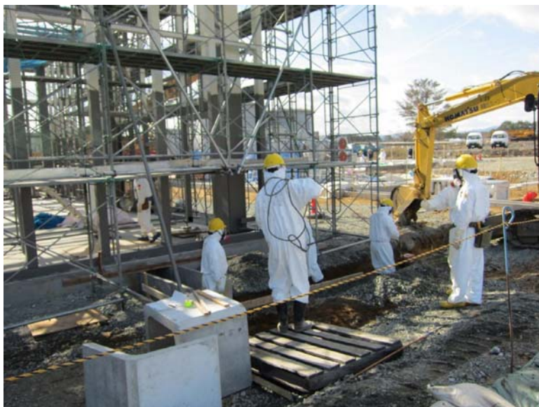
⑦-10 Construction of new switch station Jan.10, 2011 photo by TEPCO staff
