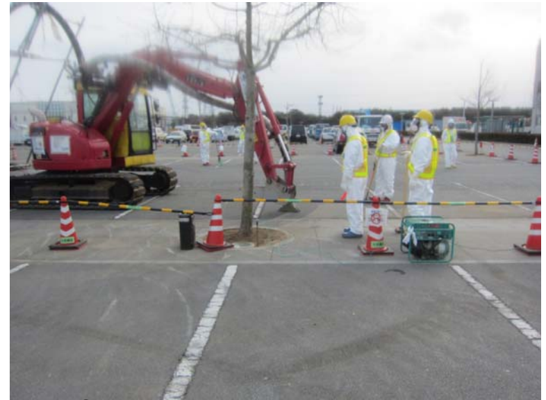
②—5 Collection work of dust and small debris at parking area of Main Anti-earthquake Building
