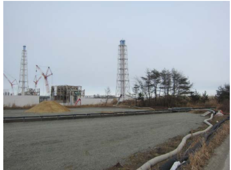
④-2 Look into Reactor Building from the hill in the southern side of Unit 4 Jan. 9, 2012 photo by TEPCO staff
