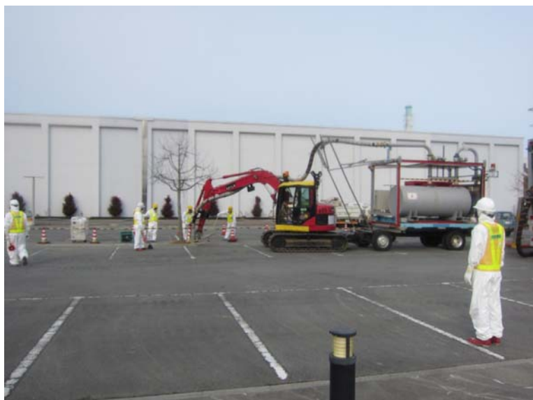
②-1 Collection work of dust and small debris at parking area of Main Anti-earthquake Building
