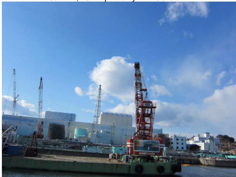
③-6 Removal of obstacle by the floating crane (from east breakwater)
