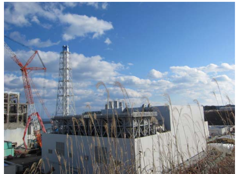
⑭— 3 Common Pool Building Jan. 14, 2012 photo by TEPCO staff
