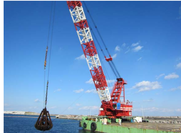
⑫ Removal of obstacle by the floating crane (from sea side yard) Jan. 14, 2012 photo by TEPCO staff
